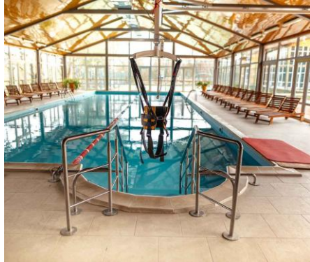
Ceiling lift for water rehabilitation of patients
